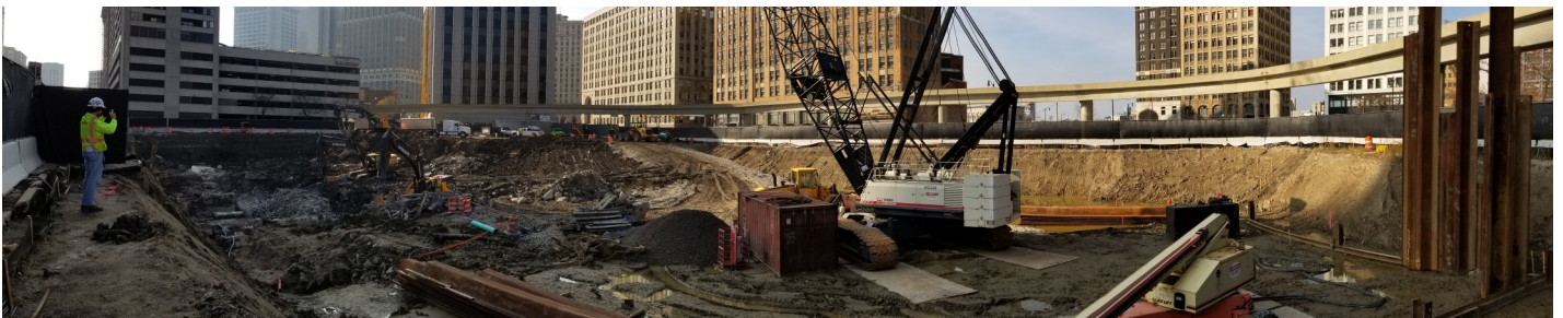
Construction site of apartment complex in Detroit, Michigan.
