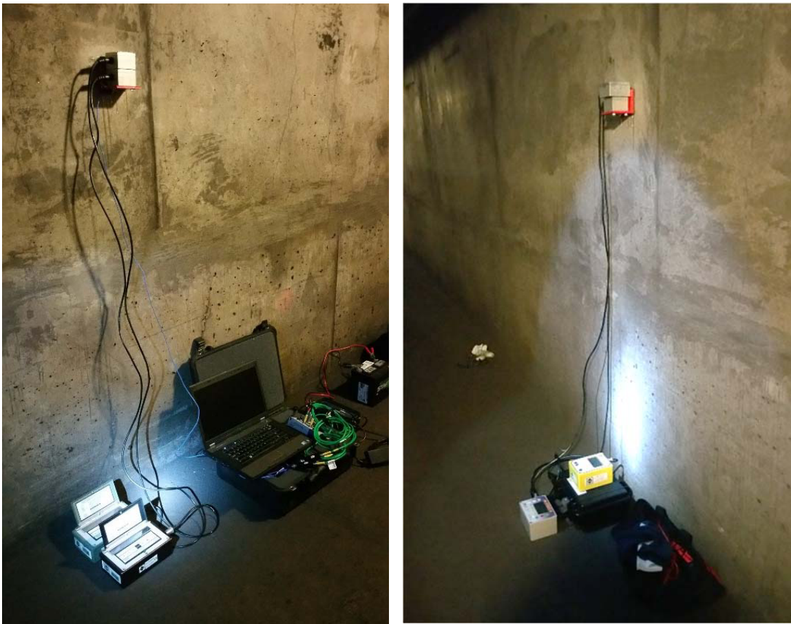
Figure 2 Gallery wall instrumentation showing velocity seismographs 5159 and 2407 and accelerometer (left) and seismograph serial numbers 7211 and 20049 (right)
